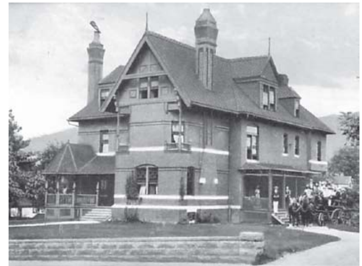
The Belmont Today parking Lot For Renaissance Hotel
